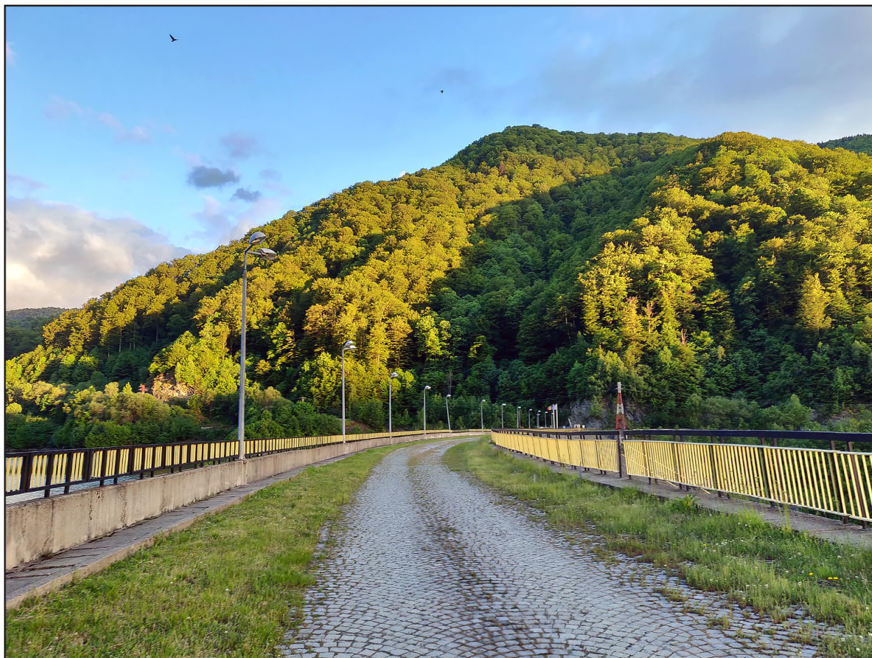
Fig. 4. Overview on the dam's crest, highlighting the pavement conditions visible at the surface.
