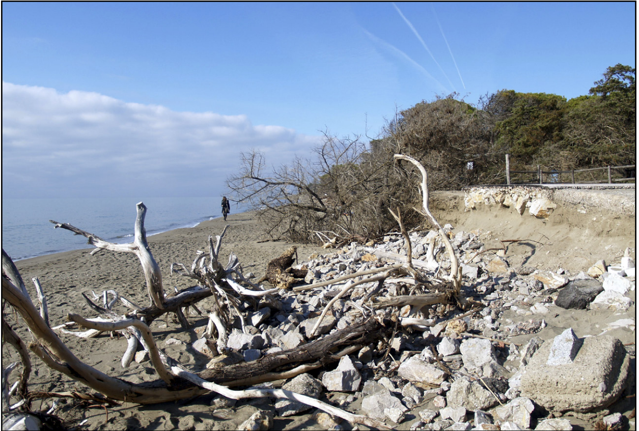
Fig. 6 Marina di Alberese: the road cut off by erosion. A parking lot and a restaurant were present in this area during the 1970s
